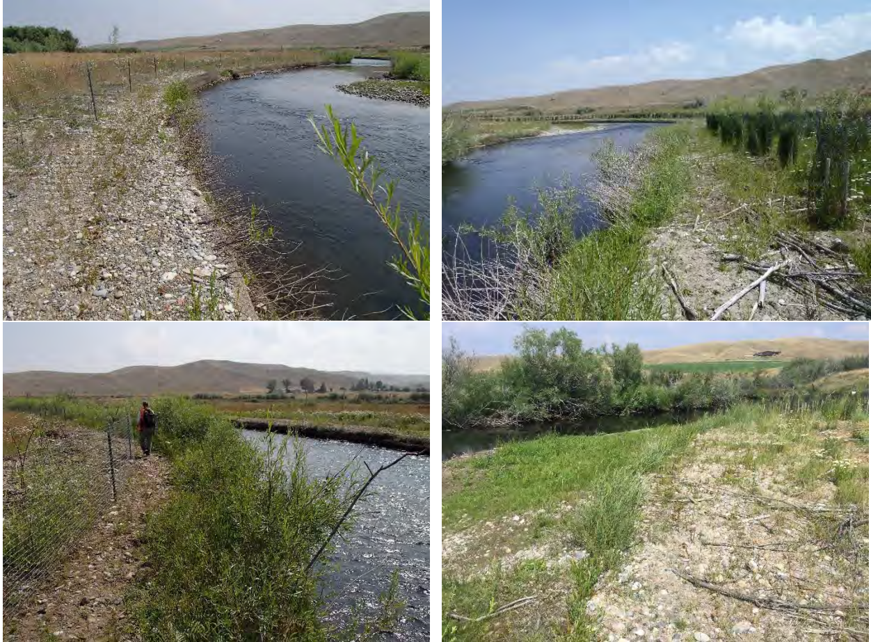
Figure 21. Top left photo of streambank treatment LB-N-7 (DVSL) Category 3 (<10%). Top right photo of streambank treatment RB-N-22 (PV) Category 2 (10 to 40%). Bottom left photo of streambank treatment LB-N-8 (PV) Category 1 (>40%). Bottom right photo of streambank RB-N-49 (BT) Category 2 (10 to 40%).
