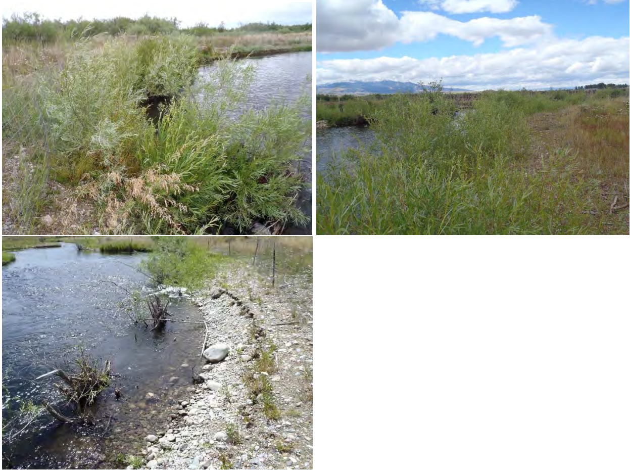
Figure 30. Top photos are of preserve vegetation (PV) streambanks showing expansion of preserved willows into the floodplain (left photo is LB-N-3; right photo is RB-N-48). Right photo is of one of the few preserve banks where erosion had occurred (LB-N-14-16).
