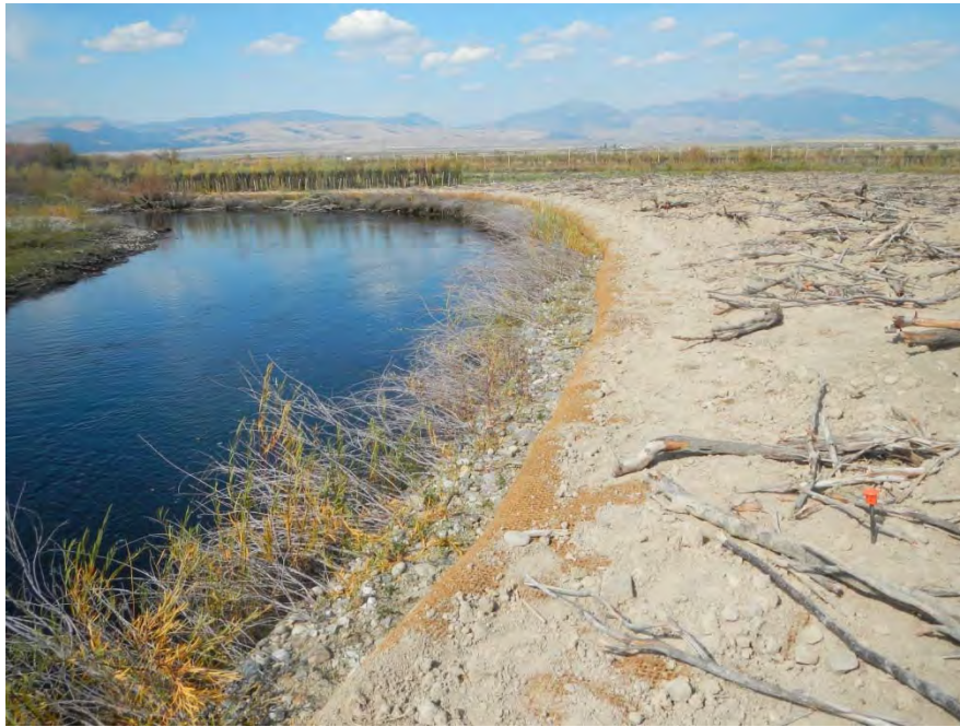
Photo 6. View downstream of bank and floodplain repairs at overflow site.
