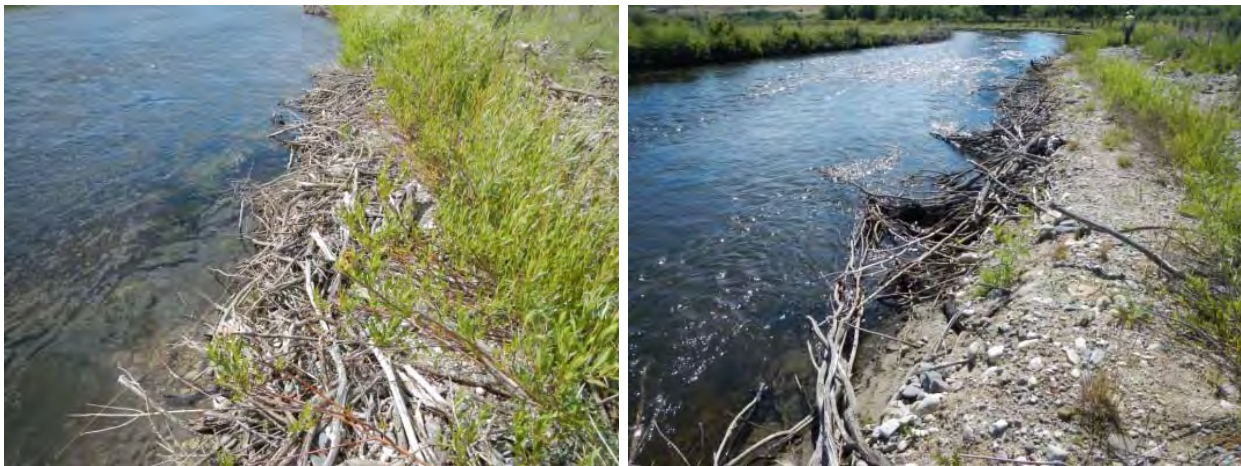
Figure 40. Left photo of brush matrix (gap) treatment with some viable brush material and right photo showing a brush matrix treatment with no viable brush material.
