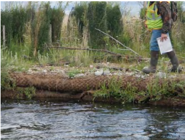
Figure 10. DVSL streambank with fabric decay and exposed coir log.
