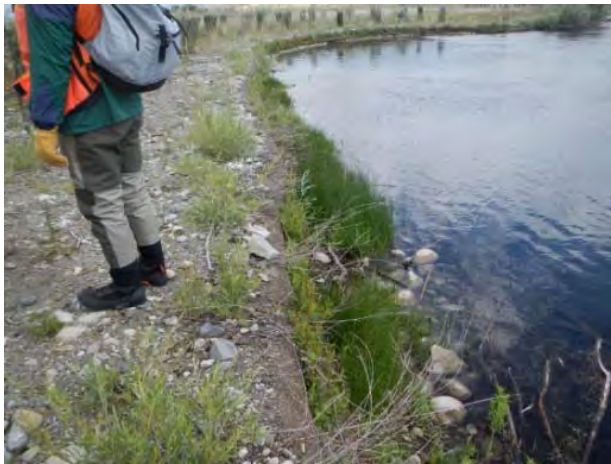
Figure 12. Colonization of wetland vegetation on toe material in front of DVSL LB-N-35.
