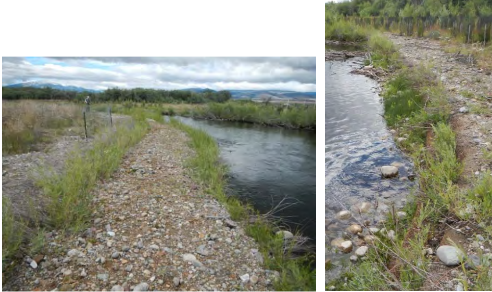
Figure 15. Bare alluvium placed behind streambank treatment.
