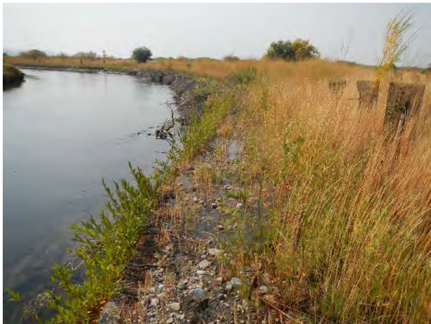
Photos 19-21. Ponding from Galen Creek beaver dams and surface water return flow into the river.
