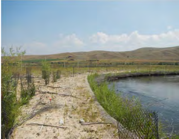
Figure 8. Bankline that was repaired following the 2014 overflow event (photo is looking upstream).
