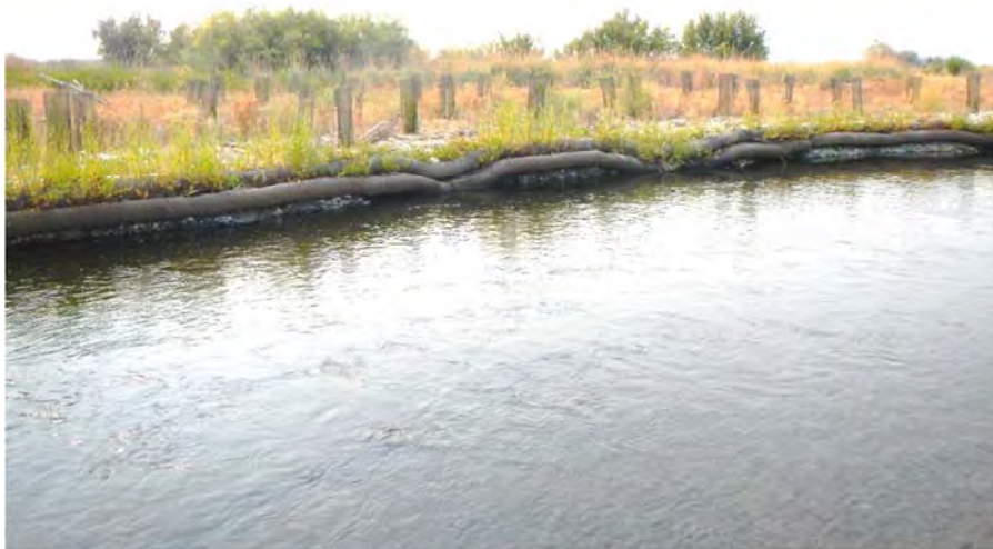
Photo 18. View downstream of bank LB-11 identified for continued monitoring.
