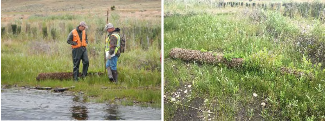
Figure 11. Coir log displaced from bank RB-N-19 and deposited on floodplain surface immediately downstream. Herbaceous wetland vegetation is growing in the coir log (right photo).
