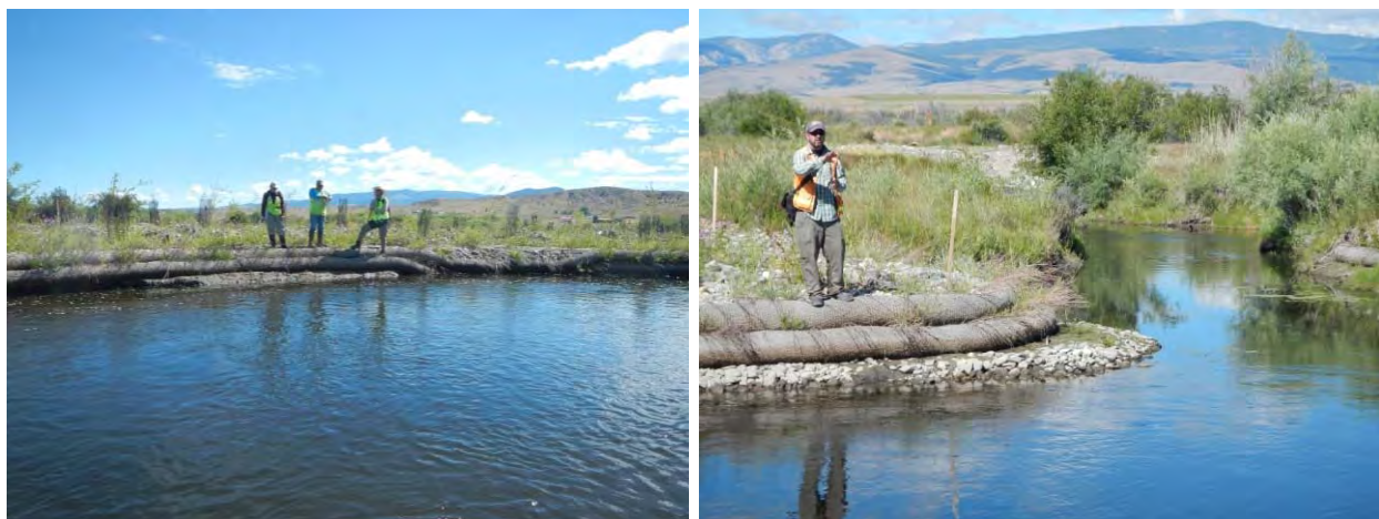
Figure 39. Phases 5 and 6 LB-46-DVSL toe loss and structure slumping (left photo) and streambank that appeared to be installed higher than Q2 (right photo).
