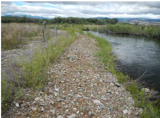
Figure 14. Willow growth in brush trench behind DVSL (LB-N-27) (photo is looking downstream).
